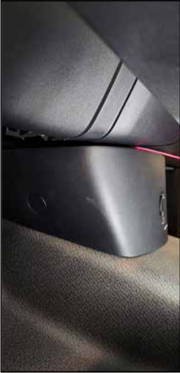
1) Wire (R2) routed above shroud to drivers side. Secure as you go.
